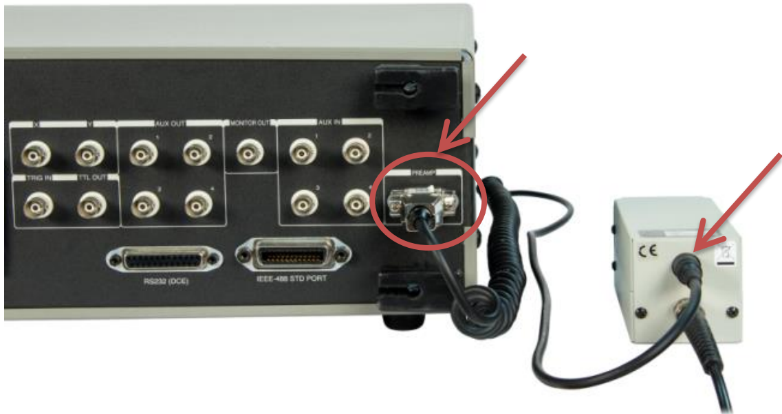
Figure 7: Amplifier Power Connection on SR810 with LIDA-Compatible Oriel Detector
